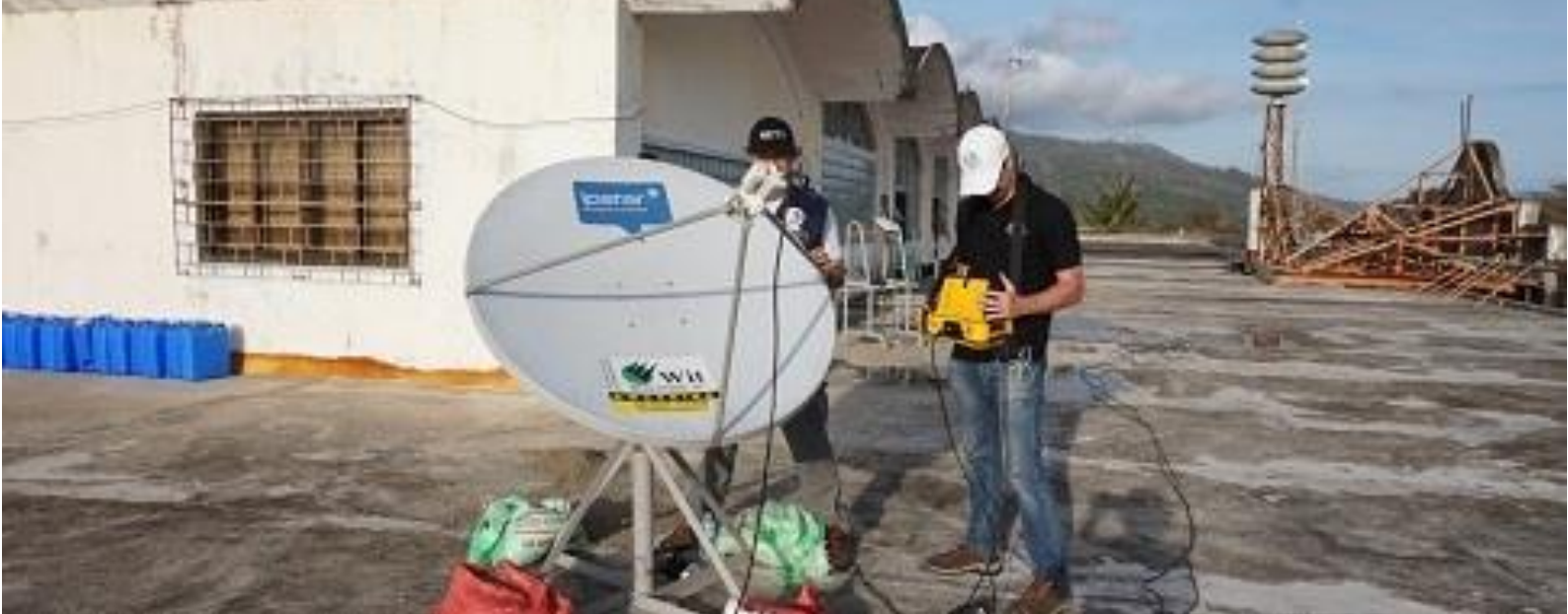
Catanduanes Island, Philippines – December 2019 Following Typhoon Kammuri, a TSF engineer installs a VSAT Internet connection for the benefit of local authorities and relief NGOs.
