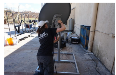
VSAT installation at first EOC at Maxwell supermarket
