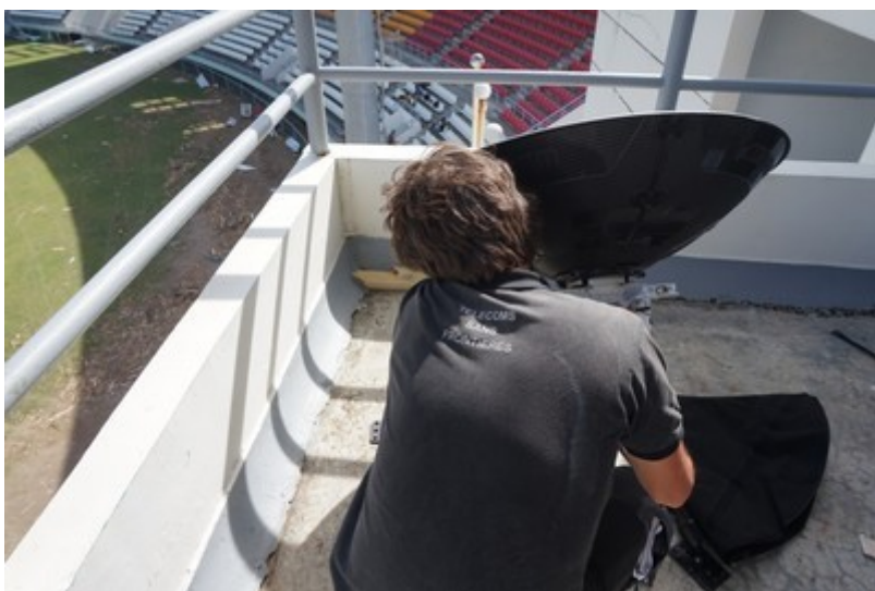
Windsor Park Stadium, Roseau – Global Xpress (GX) installation
